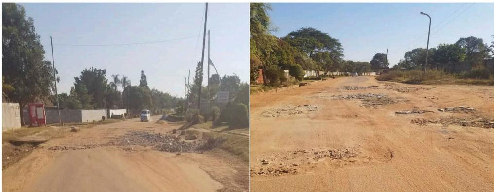
Figure 1. Concrete block debris used to fill potholes on Zambezi Road, Riverside, Kitwe.
