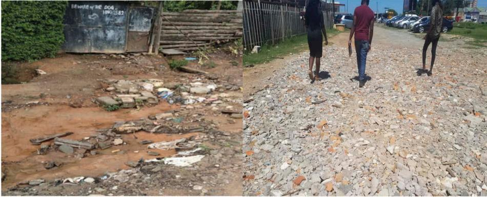
Figure 6. Construction Debris used as filling on roads in Buchi and Nkana West, respectively.
