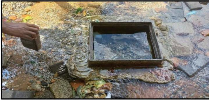
Figure 5. Leaking water valve, source, author's (2022).
