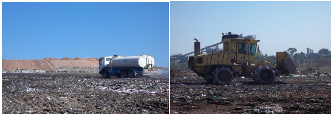
Figure 8: Water spraying and soil compaction
