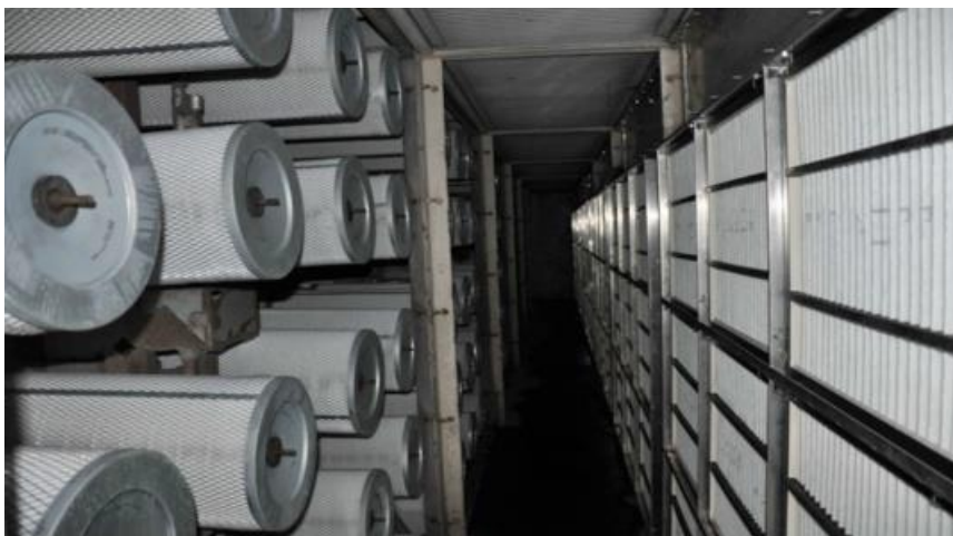
Figure 9: Filter house; Stage 1 filter to the right and Stage 2 to the left (SSE, 2012).
