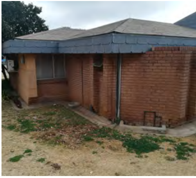
SWC asbestos roof tiles
