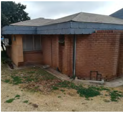
SWC asbestos roof tiles
