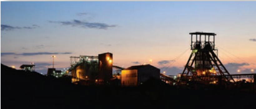
The N'Chwaning II mine headgear in the Kalahari manganese field, South Africa. (Bruce Cairncross photographer)
