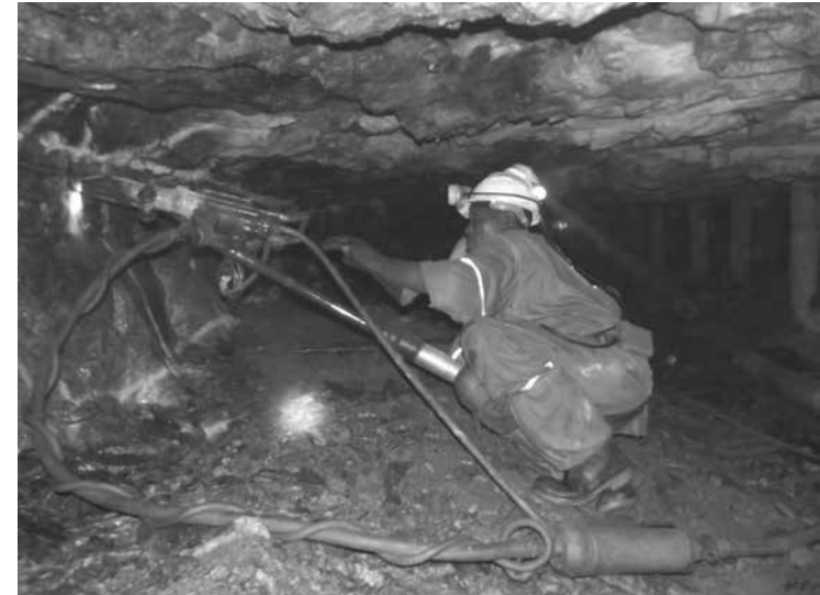
A rock drill operator at work.
