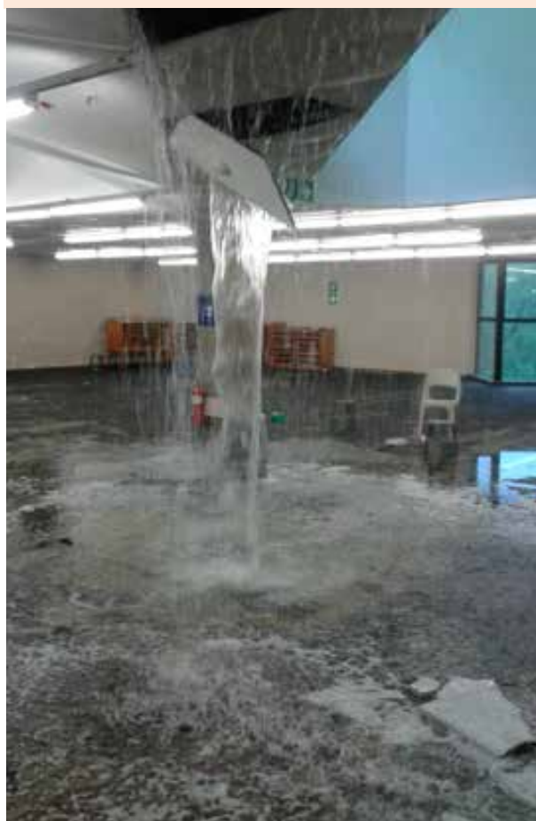
APK: Collapsed ceiling level 2
